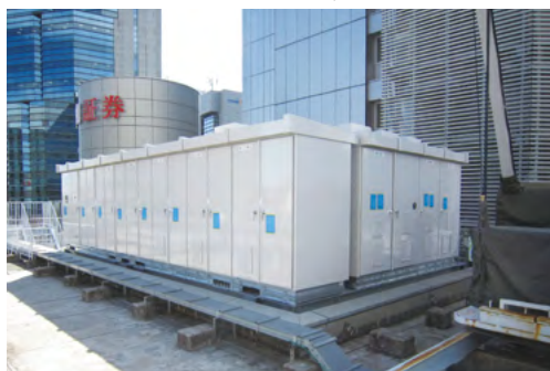
Power receiving and transforming facilities relocated to the rooftop of the Osaka branch building
